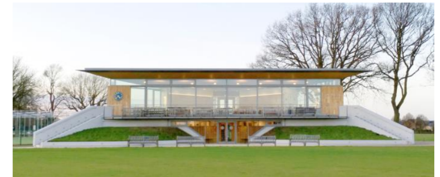
Oundle School Cricket Pavilion, East Northamptonshire, 2015
