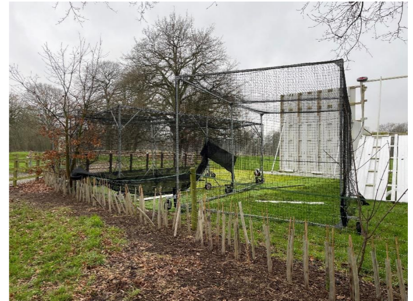
Rear nets which are in disrepair
